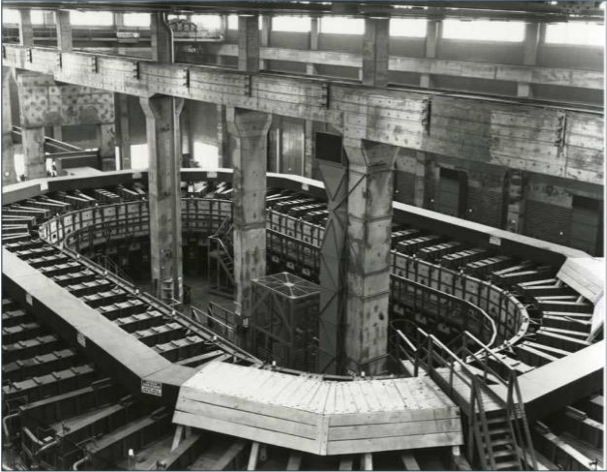
The Y-12 Electromagnetic Processing Plant's 'racetrack'. Clinton Engineer Works, Oak Ridge TN. Photo by Ed Westcott (Public domain Courtesy of Barbara Scollin)
